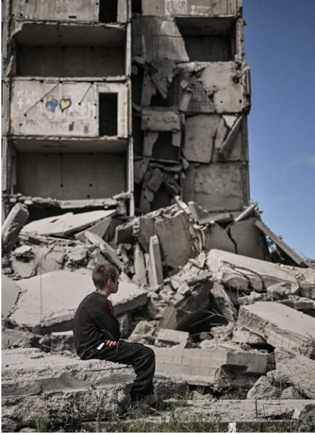
A boy sits in front of a damaged building after a strike in Kramatorsk in the eastern Ukrainian region of Donbas, in 2022. (Aris Messinis / AFP via Getty Images)
